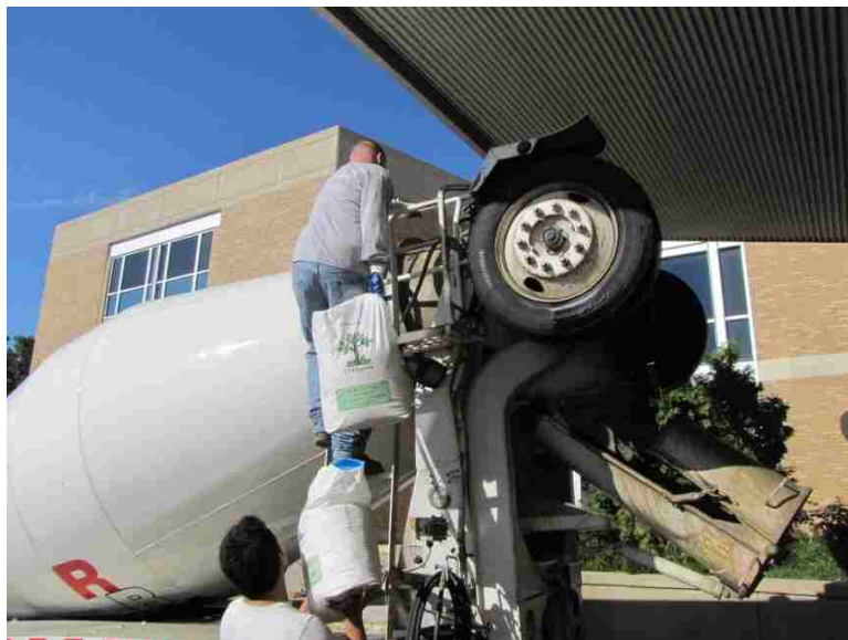
Figure 5.5 – Adding CH and Gypsum to the ready mix truck
