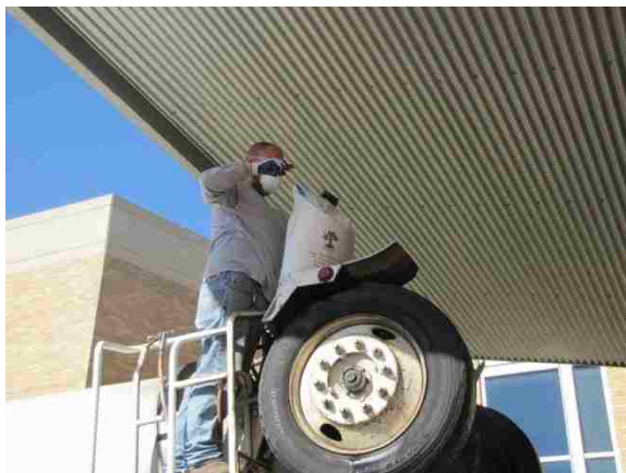
(a) Adding gypsum
