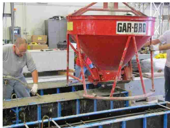
(c) Concrete placement
