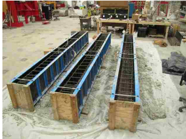
Figure 5.4 – Cages in the formwork
